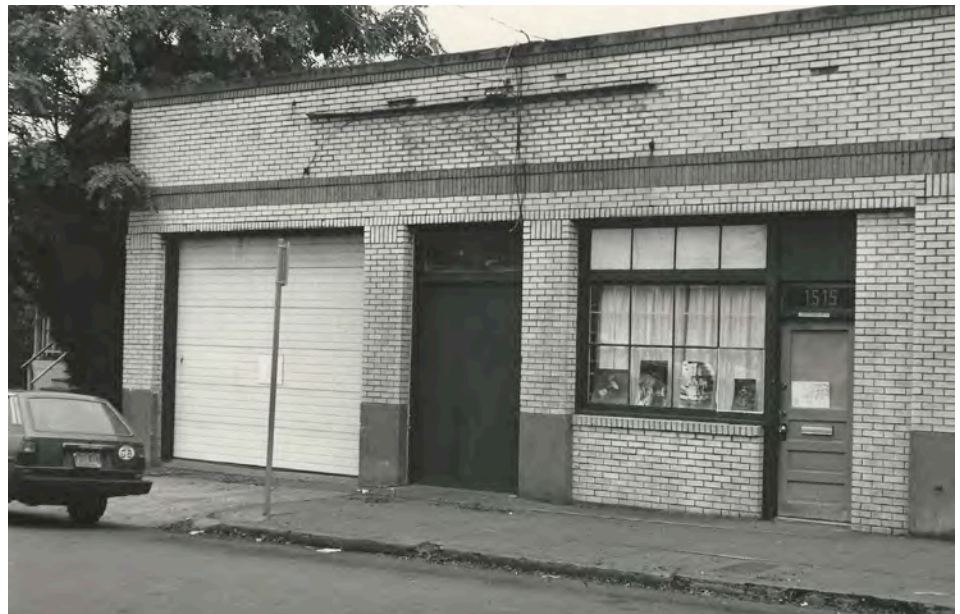
TSCO occupied a building at 1515 SE 48th Street from 1964 to 1967.
